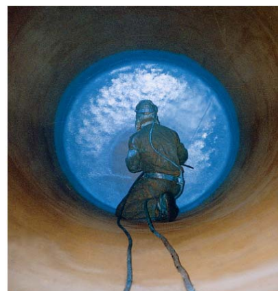
RA 564 being spray applied
