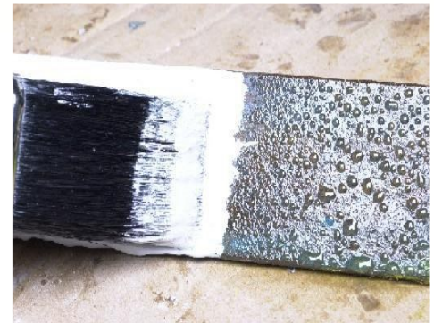
Applying RL 500PF on a wet & sweating substrate
