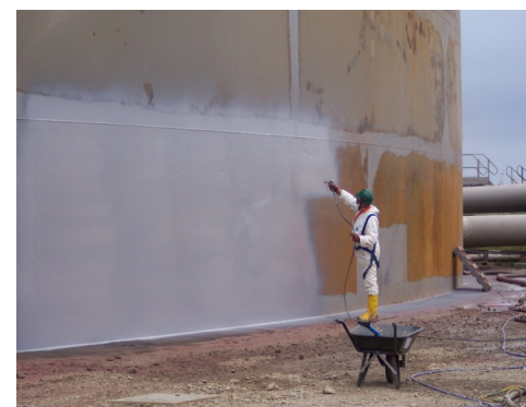
Applying RL 500PF on large tank externals
