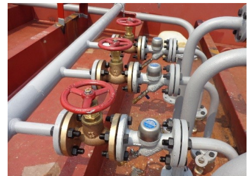
RL 500PF applied on live steam pipes
