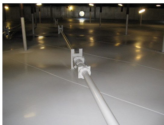
Epo-chem™ RA 500M Crude Oil Tank
