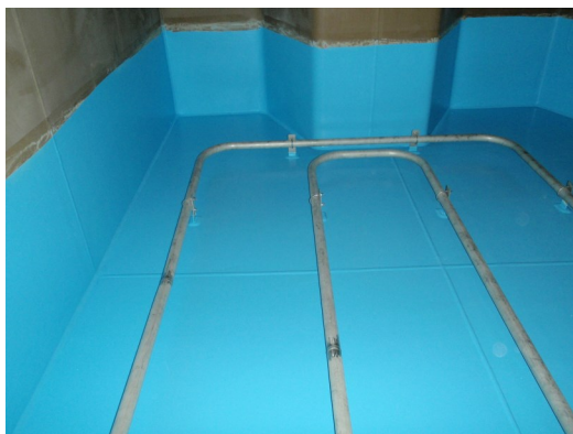
RB 364 applied in a chemical tank
