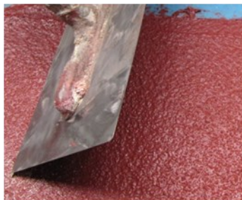
Applying InD-Cote™ by trowel
