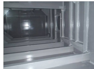
Potable Water Tank
