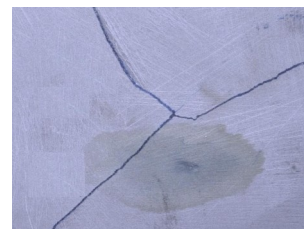
RN 800CRS Crack Repair
