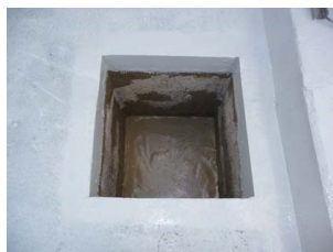
RJ 800CRS Chemical Sump Repair
