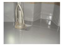
Solvent-free, rust tolerant, epoxy Novolac system offering excellent resistance to high temperatures and highly aggressive chemicals; e.g. methanol, ethanol and caustic soda.
