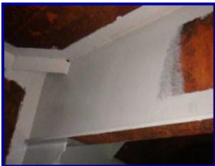
One full coat of RS 500P applied to rusty prepared steel
