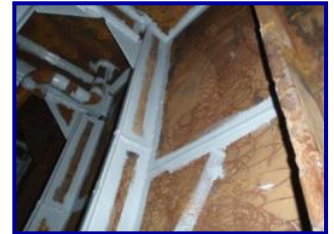
All weld areas are stripe coated regardless of their condition
