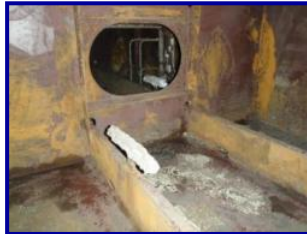
Acceptable water jetting preparation standard
