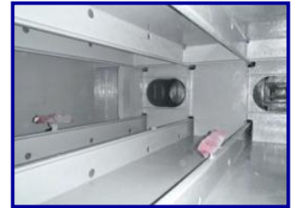
Completed application consisting of one stripe coat (RS 500P), one primer coat (RS 500P) and one topcoat (RA 500M)
