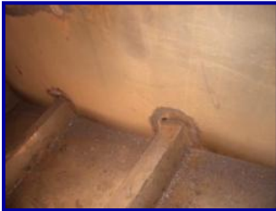
Acceptable mechanical preparation standard
