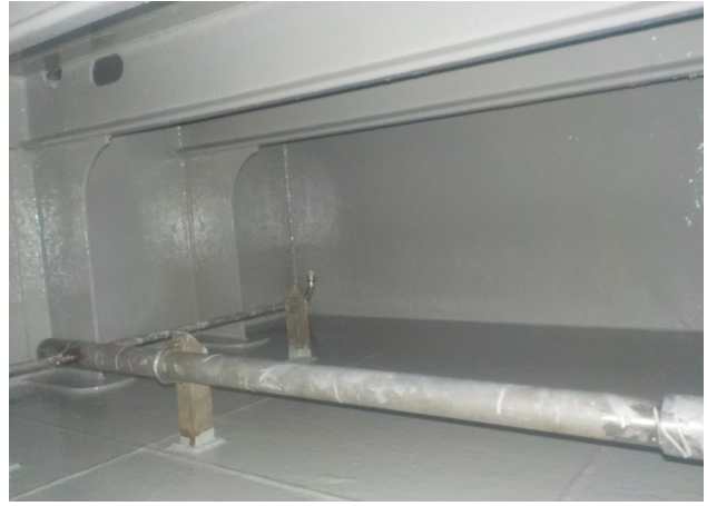
Alkali Tank Completed Application: RE 500P & RW 500
