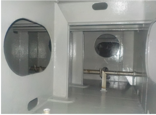
Alkali Tank Completed Application: RE 500P & RW 500
