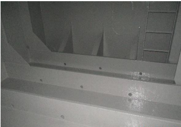
Settling Tank Completed Application: RS 500P and RA 500M
