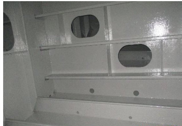
Settling Tank Completed Application: RS 500P and RA 500M
