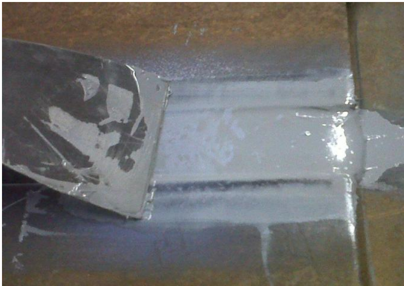
10mm mild steel plate, gap prepared by hand grinder and Ceram-chem™ RH 500 putty applied with a spatula.
